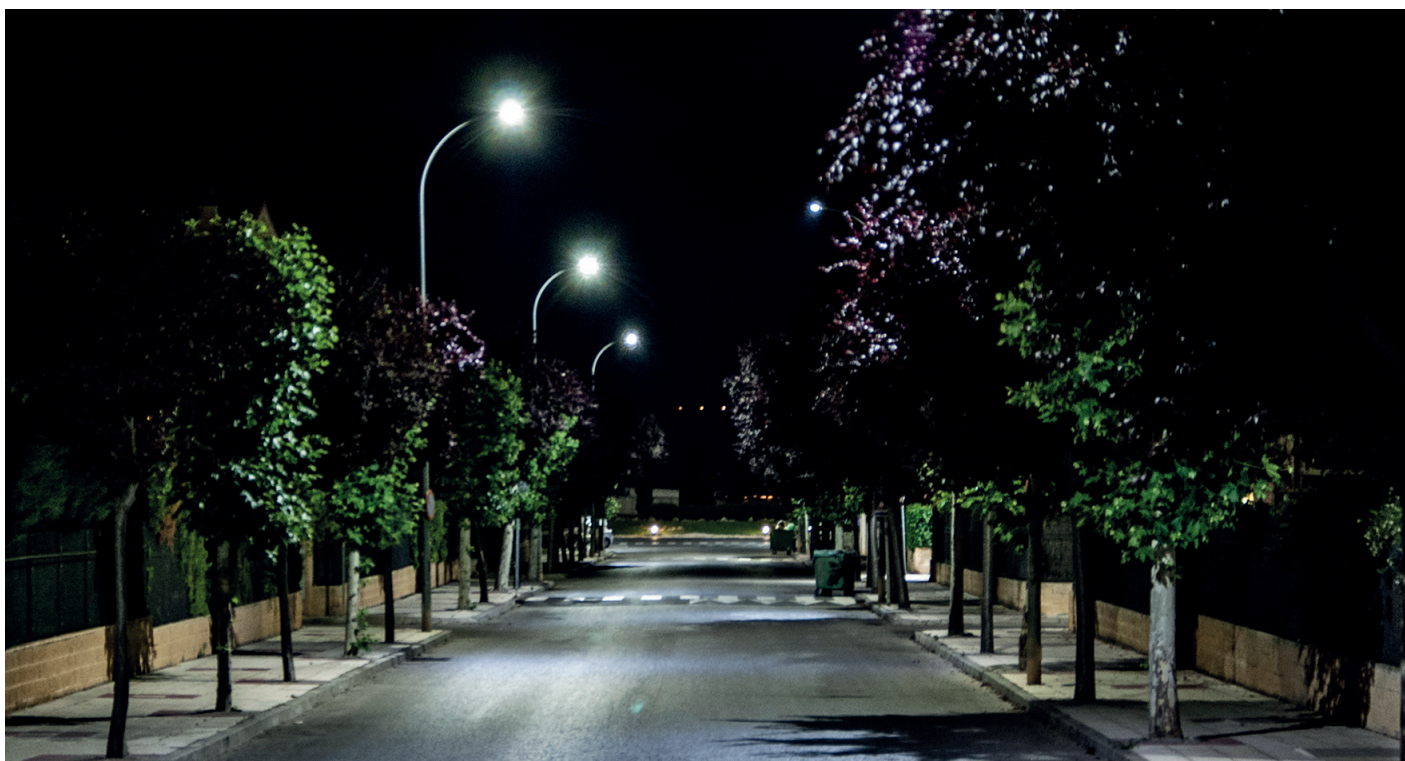
Street lighting 📍 Alovera (Guadalajara)
