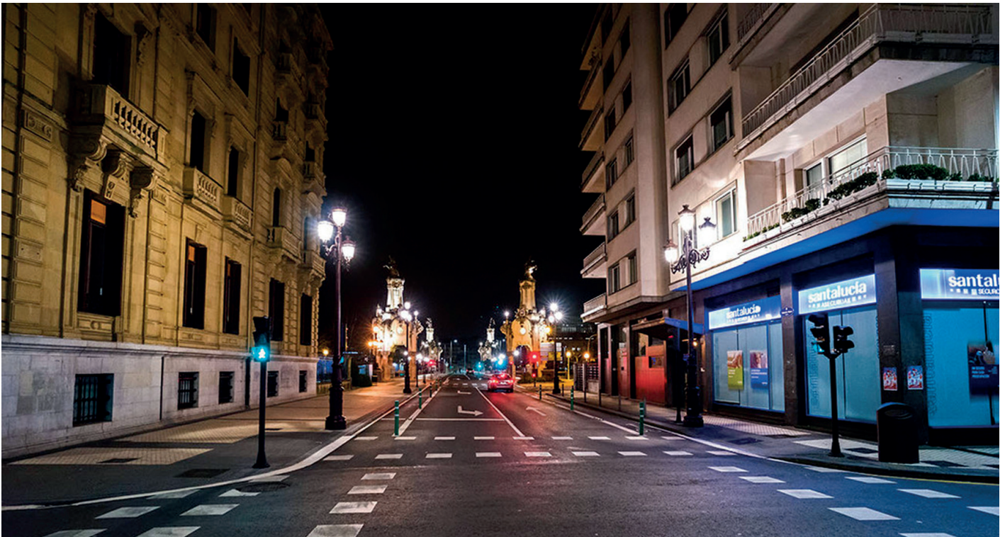
Sensorization of the street lighting 📍 Andoain (Guipúzcoa)
